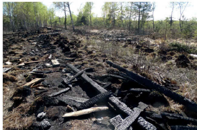
Sudegusi medinio tako dalis Wooden part of the path damaged by fire
