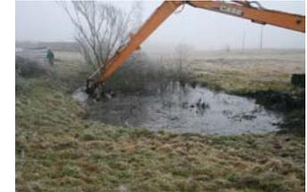
Mud removal should be performed as the pond loses its esthetic and functionality
