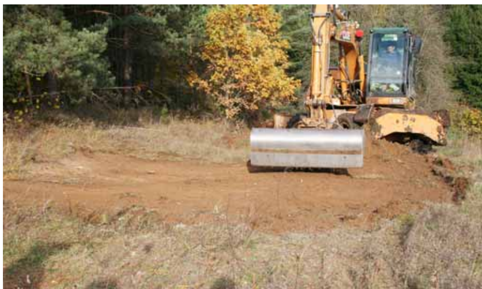
Removal of upper vegetation layer in nesting site
